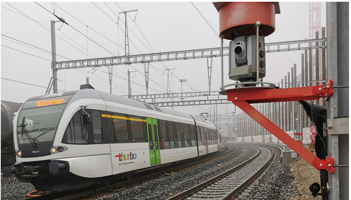
Trimble S7 total station with the construction site for the renovation of the railroad station in Wil (Canton of St. Gallen, Switzerland) in the background
