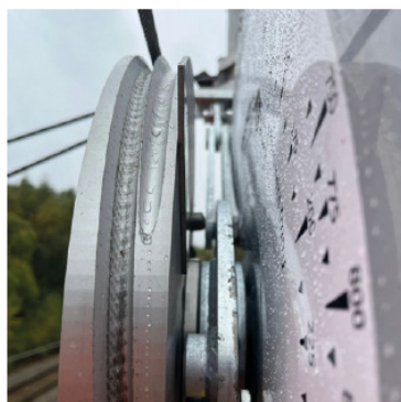
Installation on Sheffield tram 2024
