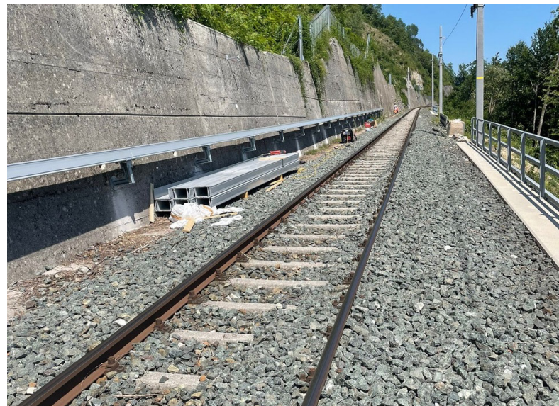
ARCOSYSTEM® safely attached to a slanting concrete wall with the aid of the system's supporting range of bespoke steel bracketry
