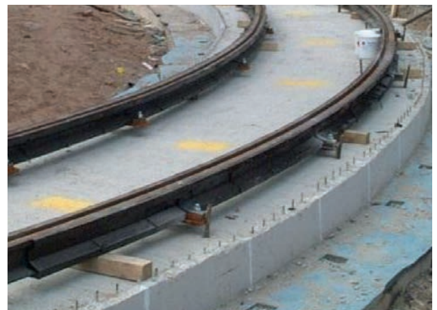
Pre-Coated Rail Track Under Construction
