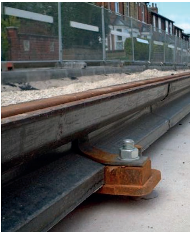
Installation of Pre-Coated Rail
