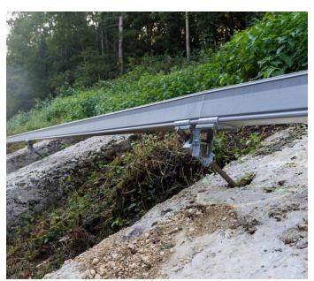
The run of troughing attached to the rock face with the aid of ClickFit brackets
