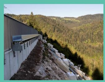
The composite troughing can be fastened to a variety of trackside structures, such as ballast boards and railings here during an installation in Germany's Black Forest
