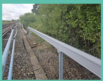
The flexible ARCOSYSTEM® troughing can be easily adjusted for height and directional changes during a long run
