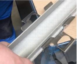
Slotting the troughing into place, activating the bracket to 'click' shut
