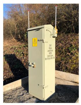
The trackside cabinet houses the transmitters, axle counters and control unit of the permanently installed warning system
