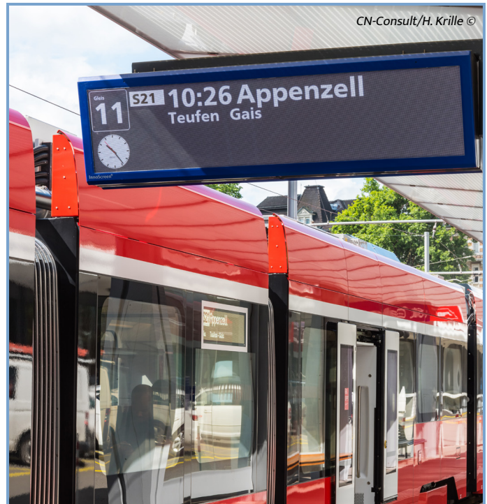
Display technology has improved over the years with both LED and TFT displays offering a wide range of possibilities to inform the passenger at the station
