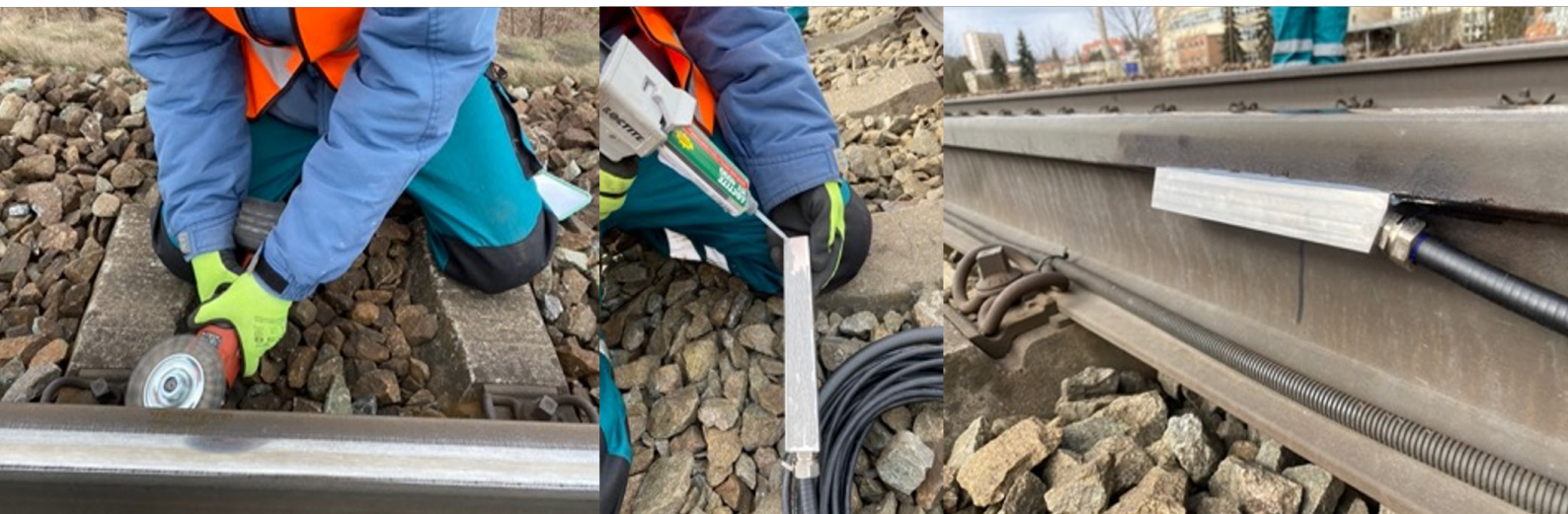
Installation of DXMD and DACT
