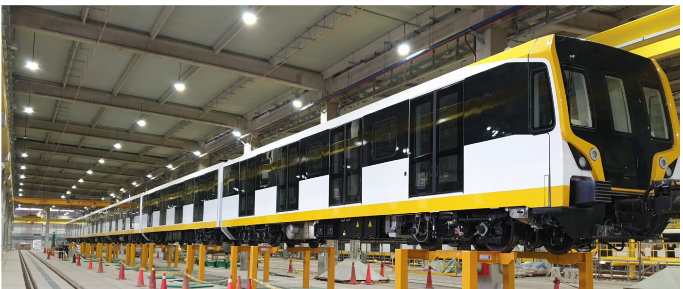
Underfloor lifting system for heavy trains with up to seven carriages and a length of 120m
