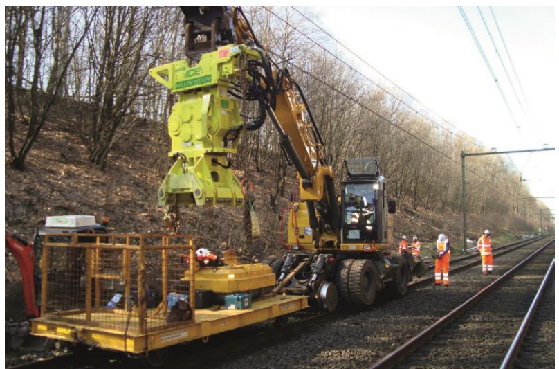
Figure 2: Road-rail excavator with attached vibration unit.
