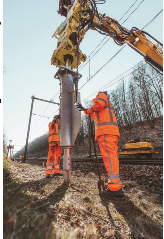
Figure 3: First process step: Align and insert guide pin.
