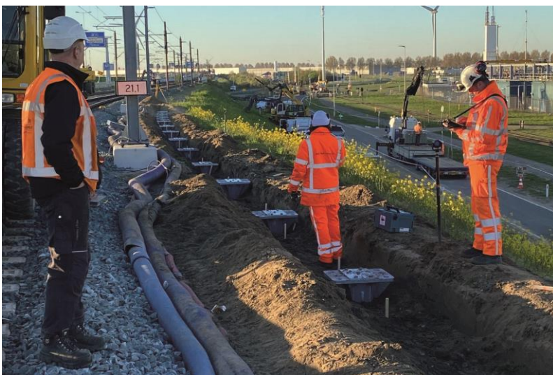
Figure 5: GSF-foundations for noise barriers at project Theemsweg in Amsterdam
