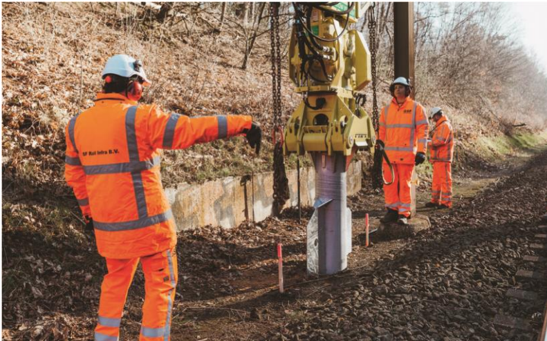
Figure 4: Second process step: Inserting the soil shield
