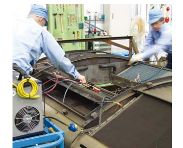
Train air conditioning system
