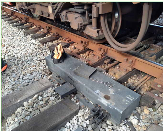
Signalling cable fixation with box Brazil
