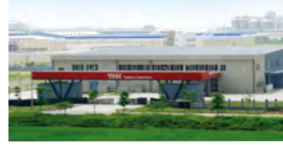
● THK MANUFACTURING OF VIETNAM CO., LTD. Site: 19,553m 2 (210,466sq.ft.) / Floor space: 23,525m 2 (253,221sq.ft.)
