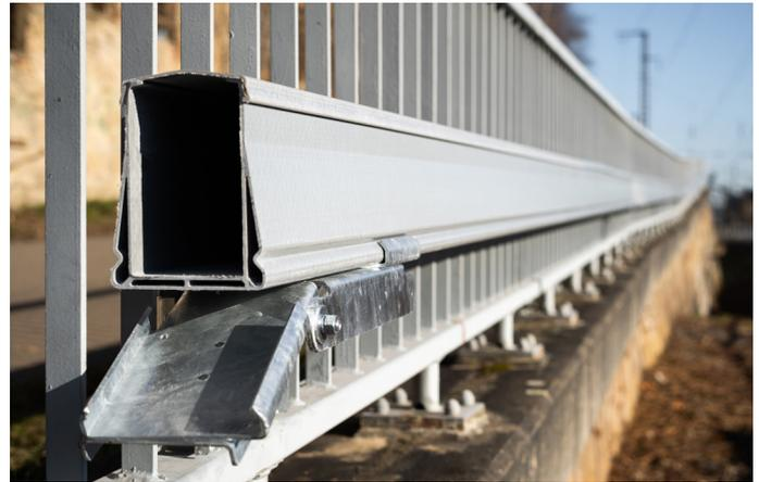
serving as roadside barriers as the route led to the railway station in town. The images of the job show just how adaptable ARCOSYSTEM® can be, and how the bespoke range of brackets can secure the troughing to a variety of surfaces.
