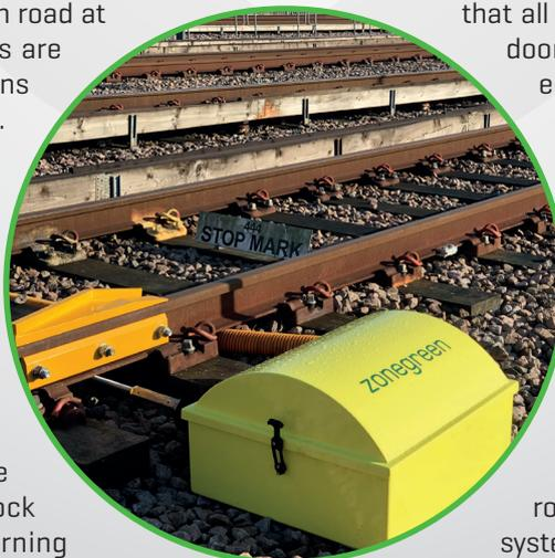
system, lowering derailer and setting inbound/outbound shunt signals [6].
