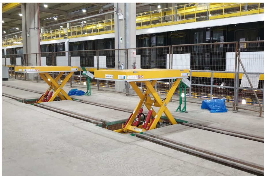
In the service area, hydraulic lifting tables lift loads of up to two tonnes (underfloor axle racks)
