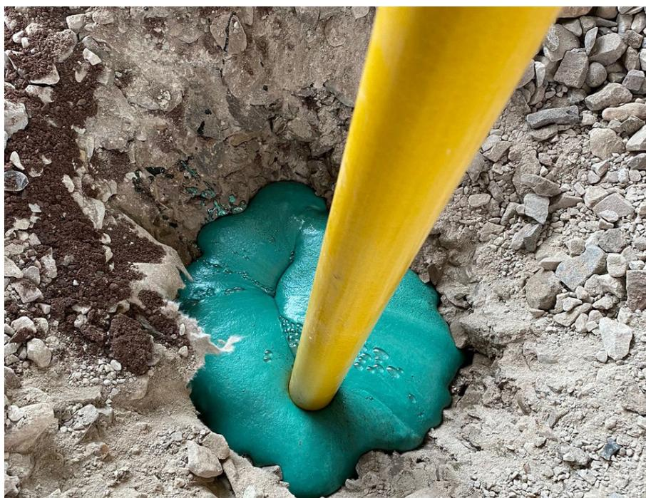
times its initial volume to create a lightweight, high-density foam. That foam mixture rises to fill the hole and encapsulates the post, becoming a solid mass able to hold the post within ten minutes. Curing time is 24 hours but the post is hard enough to fix to within one hour.
