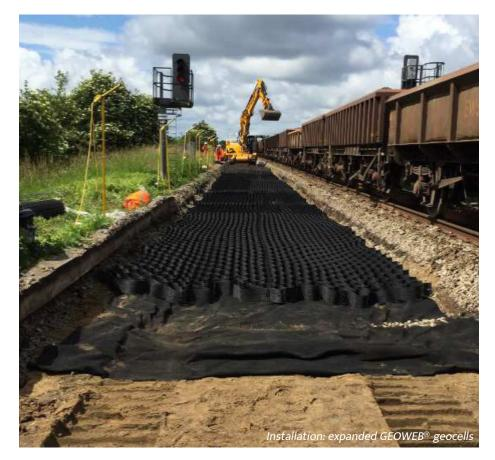
Network Rail has approved the GEOWEB® Soil Stabilisation System as the solution in areas with soft soils to improve and regulate track bed stiffness, while reducing maintenance, installation time and cost.
