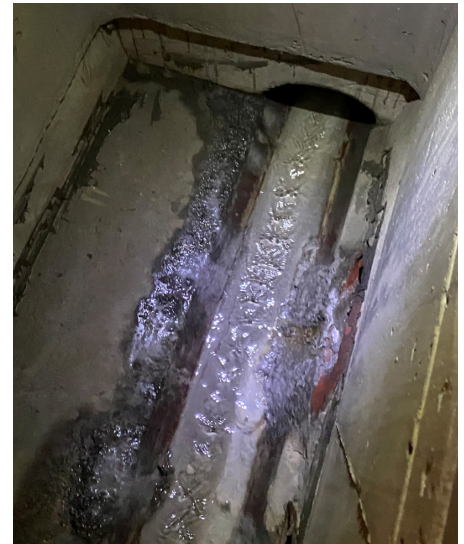
2 months after water jetting
