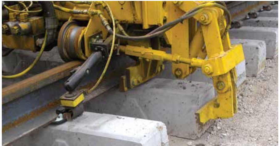
Clipping is carried out by a Nipper-Clipper mechanism on the New Track Construction Machine.
