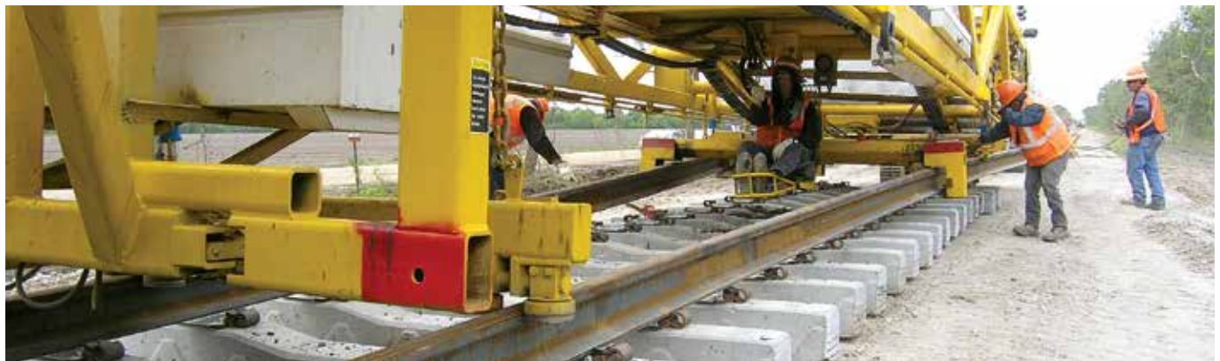
Rail Guide rollers suspended from the Laying Beam. Rails are guided into place on ties by an operator positioned below the beam.
