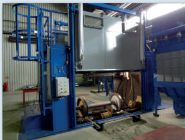
A wheelset in a drive through cabinet
