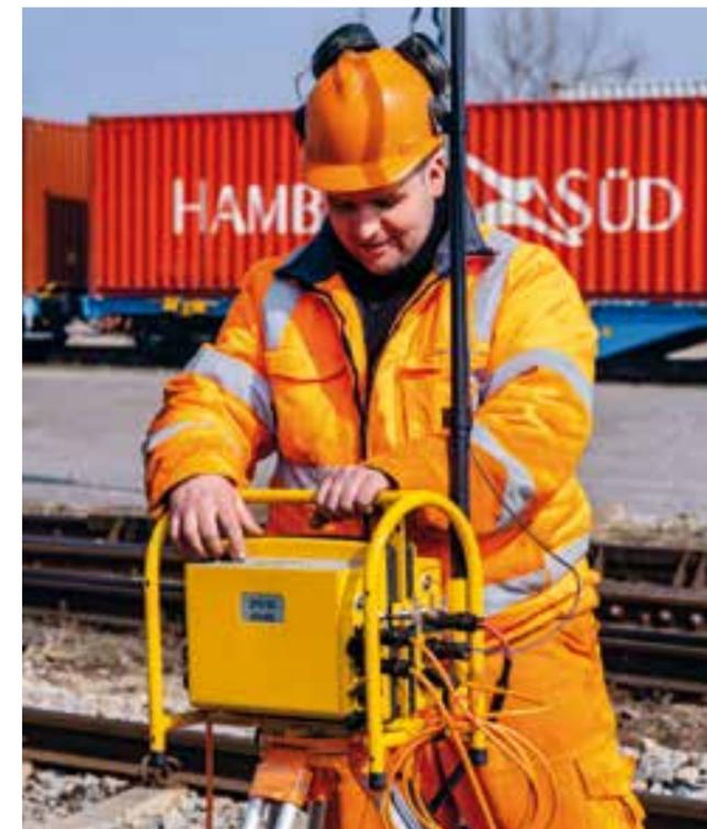
**Fig. above** The activation point for automatic train detection is composed of the wheel sensor F500-SEN, the connection box F500-AB and the radio transmitter ZFS.
