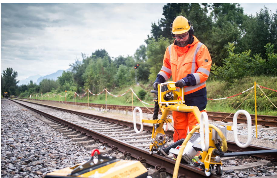
Picture 3: Due to its hybrid drive concept, the 13.49 rail head grinding machine is half as heavy as common grinders and delivers accurate pattern in less time © Robel
