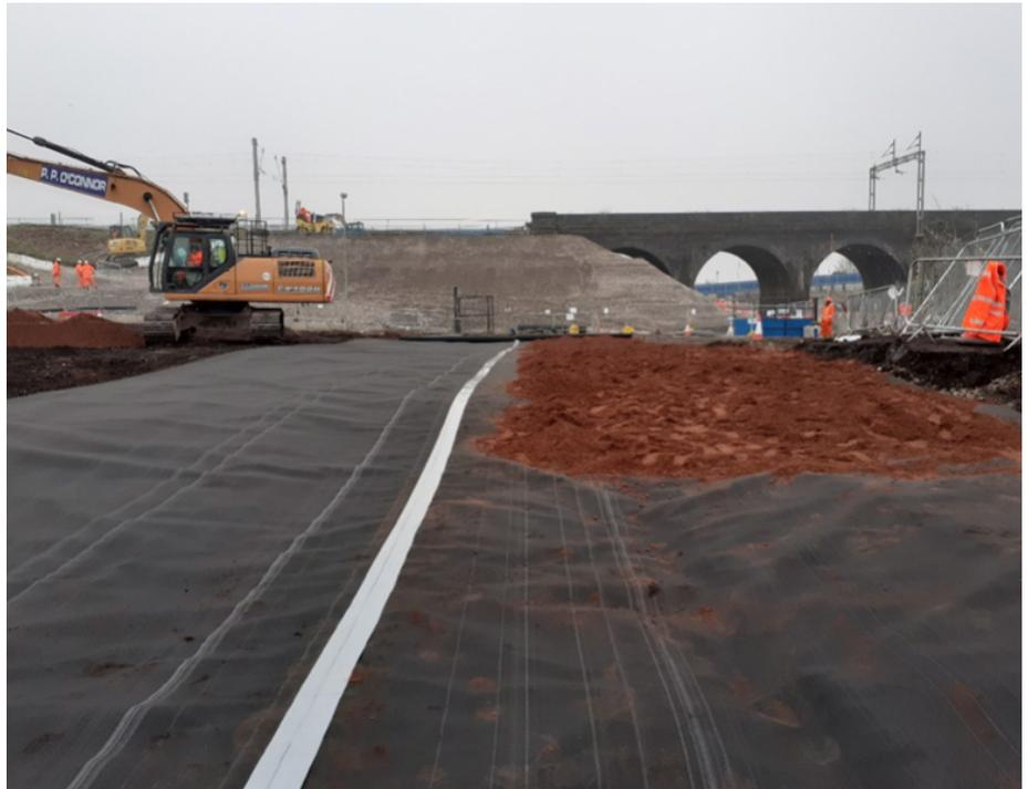
With strict guidance in place, regarding the mapping and treating of knotweed, Network Rail has traditionally used pesticides and herbicides to treat the problem. CuTex, however, is a more effective solution that only has to be laid once, as opposed to repeated cycles with chemicals.
