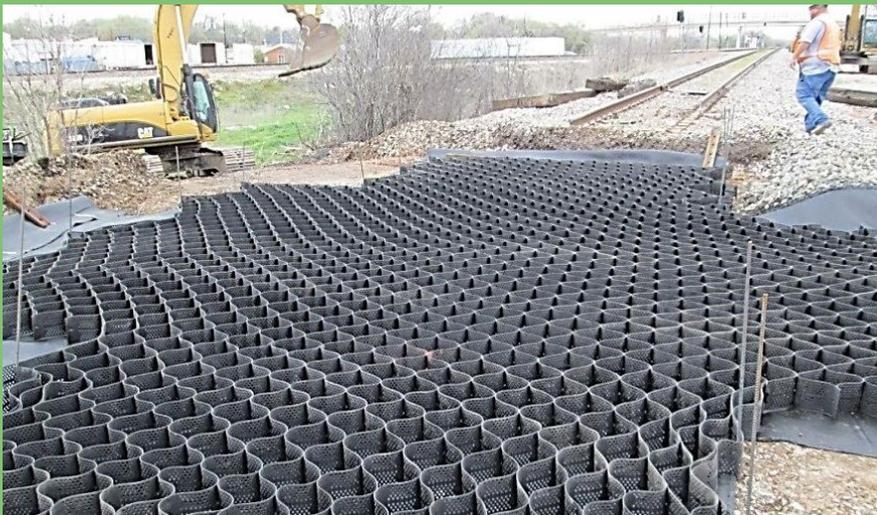
Offering the ability to repair washouts and address localised track issues quickly and economically with a single solution, the GEOWEB geocells have gained acceptance by the rail industry as
