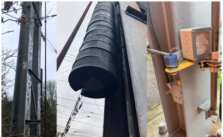
Balance Weight Monitoring Device in use in Bedford for Network Rail.
