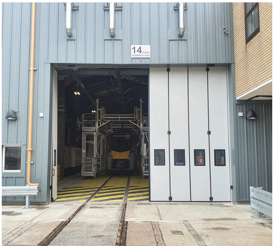
A recent installation at Crown Point Depot – Road 14 in Norwich. One set of Osprey folding doors for an opening 6.5m wide by 5m high. The door is electrically operated with four leaves folding to each side.
