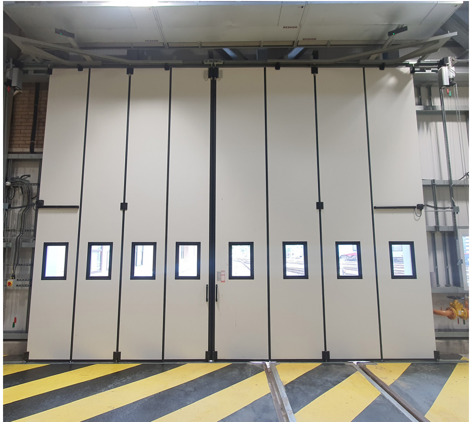
A recent installation at Crown Point Depot – Road 14 in Norwich. One set of Osprey folding doors for an opening 6.5m wide by 5m high. The door is electrically operated with four leaves folding to each side.
