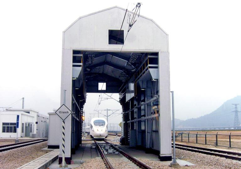
Check Point / Tunnel, installed at the trackside, consists of many modular function units, and is designed to carry out various inspections and measurements for a moving train. This includes monitoring of the wheel profile, detection of wheel cracks by ultrasound, measuring of brake pad and pantograph carbon strip, as well as fault recognition for other visible key components, such as lost bolts, adhering foreign objects by machine vision.
