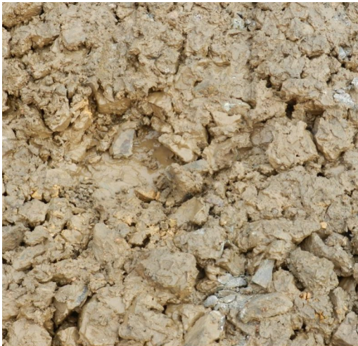
Figure 11. Slurred formation at Bradley Junction, prior to laying Geocomposite Microporous Filter
