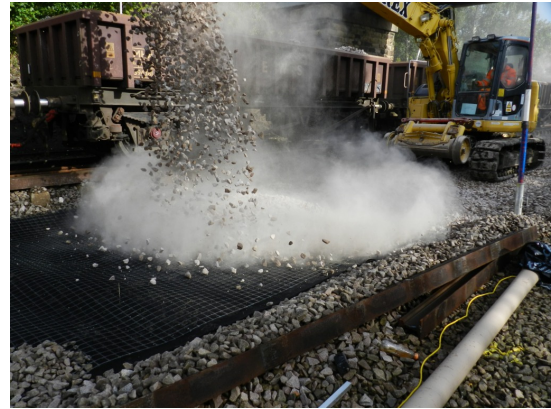
Figure 12. Geocomposite Microporous Filter Installation
