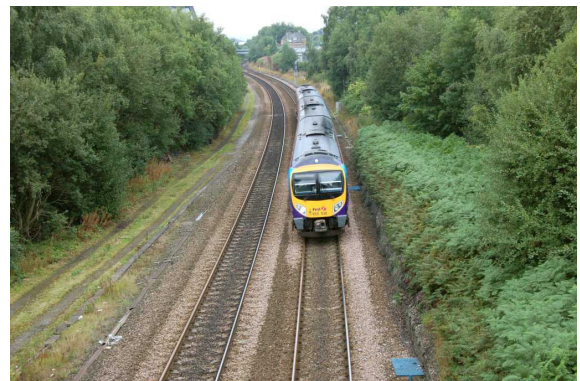
Figure 13. Bradley Junction Installation as of Today
