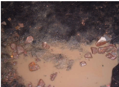
Figure 8. Top of Geocomposite After 70 Million Gross Tons of Loading
