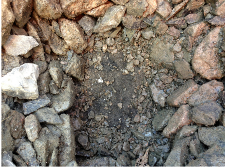
Figure 14. Test Pit at Bradley Junction - After Reconstruction with Geocomposite Microporous Filter
