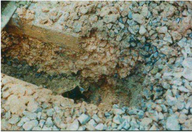
Figure 2: Severe subgrade erosion
