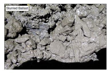
Close up of SP1 shows that where no Tracktex is present, formation failure is evident.
