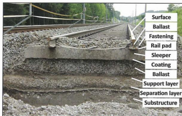
Fig. 1: Example of a modern, multi-layered ballast bed
