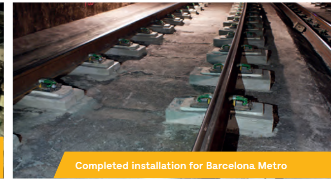
Lightweight concrete block delivered pre-assembled
