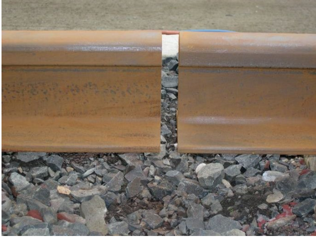
Figure 7: Rail ends cleaned - Correct
