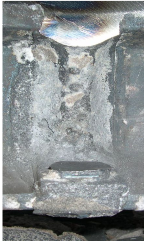
Figure 19: Weld with too short reaction time
