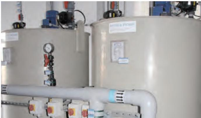
The wastewater toilet tanks of the aircraft have to be flushed with a disinfectant solution ("blue water"). The preparation of blue water is done by using a concentrate and fresh water.
