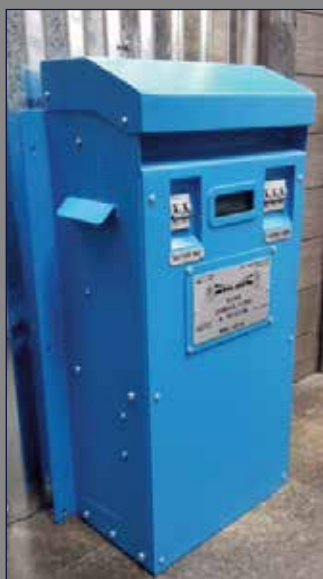
Locomotive Layover Battery Charger 480VAC / 575VAC to 74VDC
