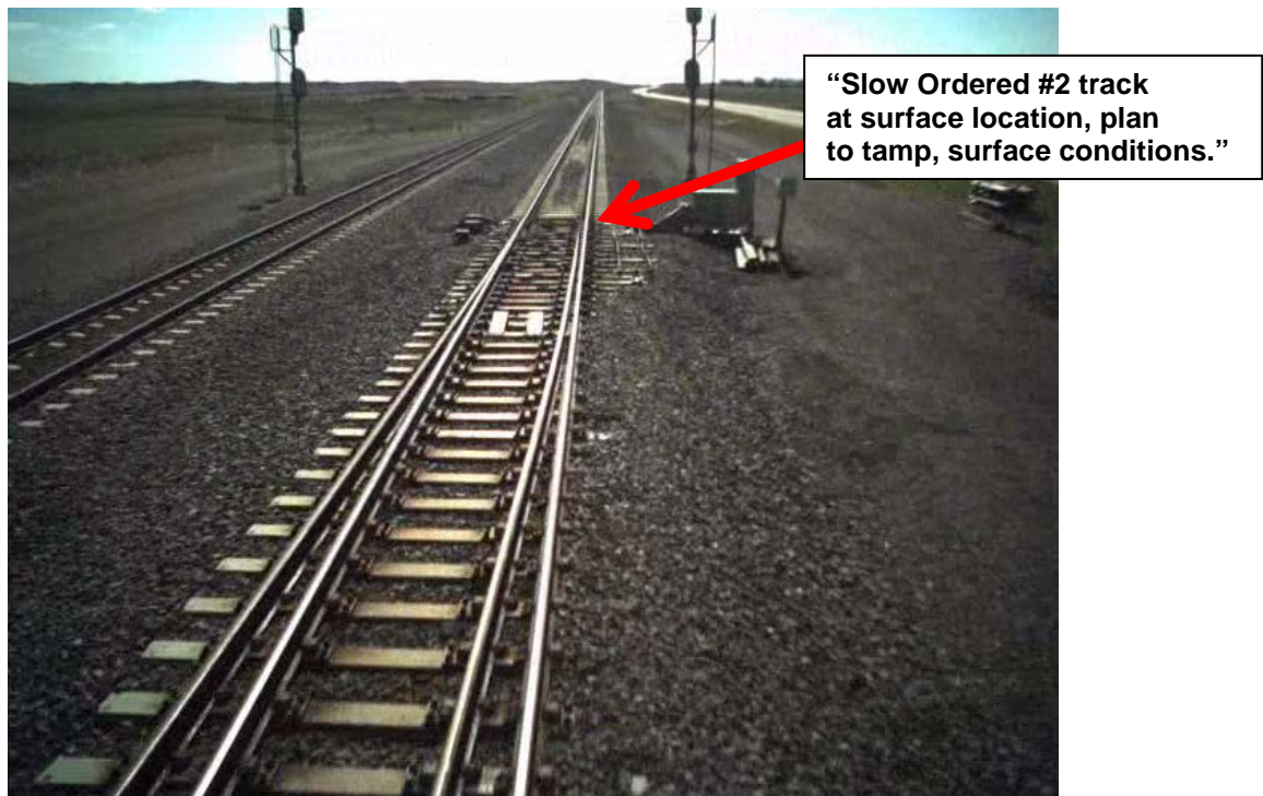
Figure 6. Example combo cluster inspection findings and remedial actions. Photographs from Union Pacific Evaluation Car (EC) Right of Way Video. Comments from field personnel.
