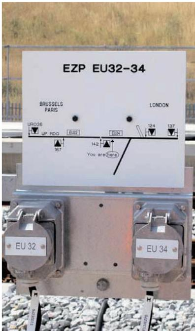
Figure 4 - Engineering Zone of Protection (EZP) Module
