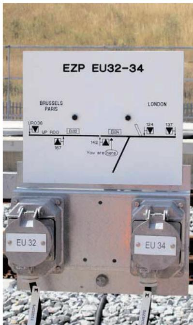
Figure 4 - Engineering Zone of Protection (EZP) Module
