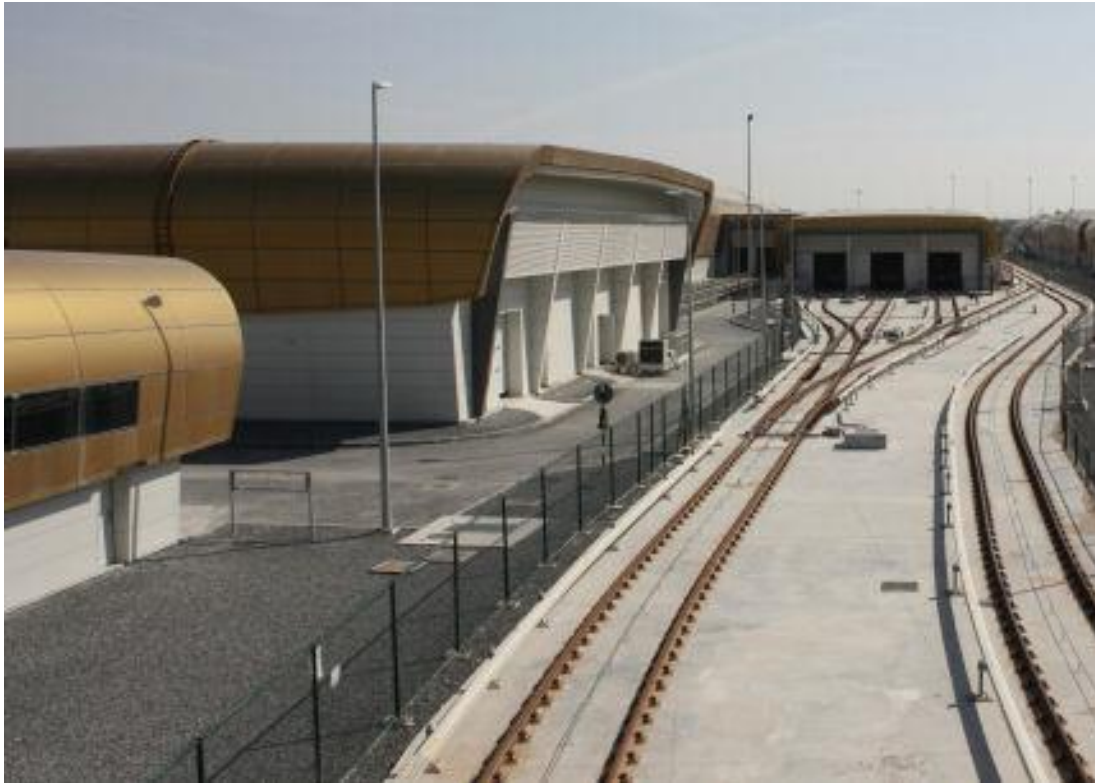
Fig 3: Dubai Metro Maintenance Depot
