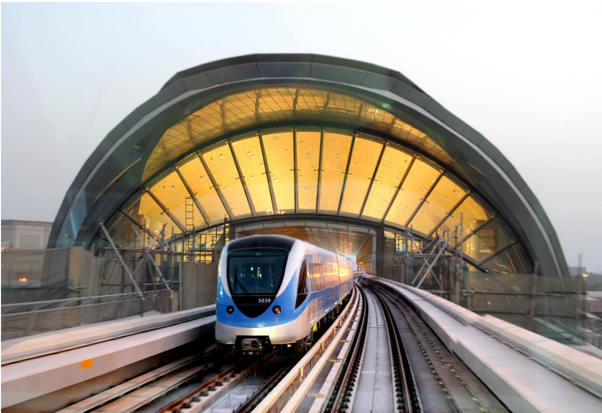
Fig 1: Dubai Metro – Driverless Trains
