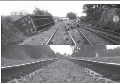
UK: Cause of cyclic top condition which caused derailment (shallow formation) was not addressed.
