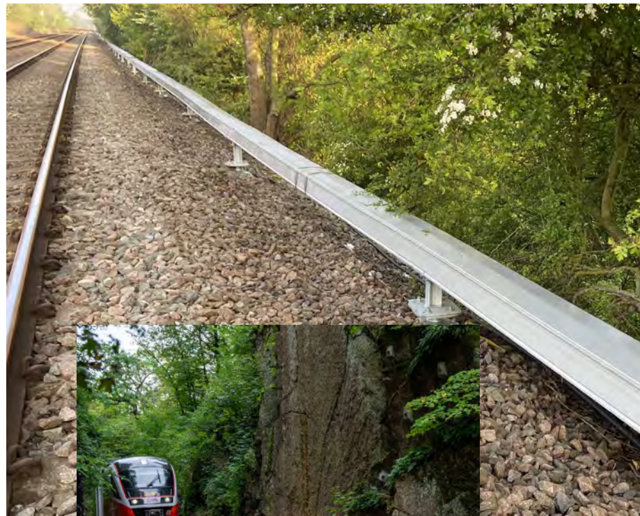
ARCOSYSTEM® installed via the 'Rapid Route' method with ground-screwed Anchor Screws, near Castleford
