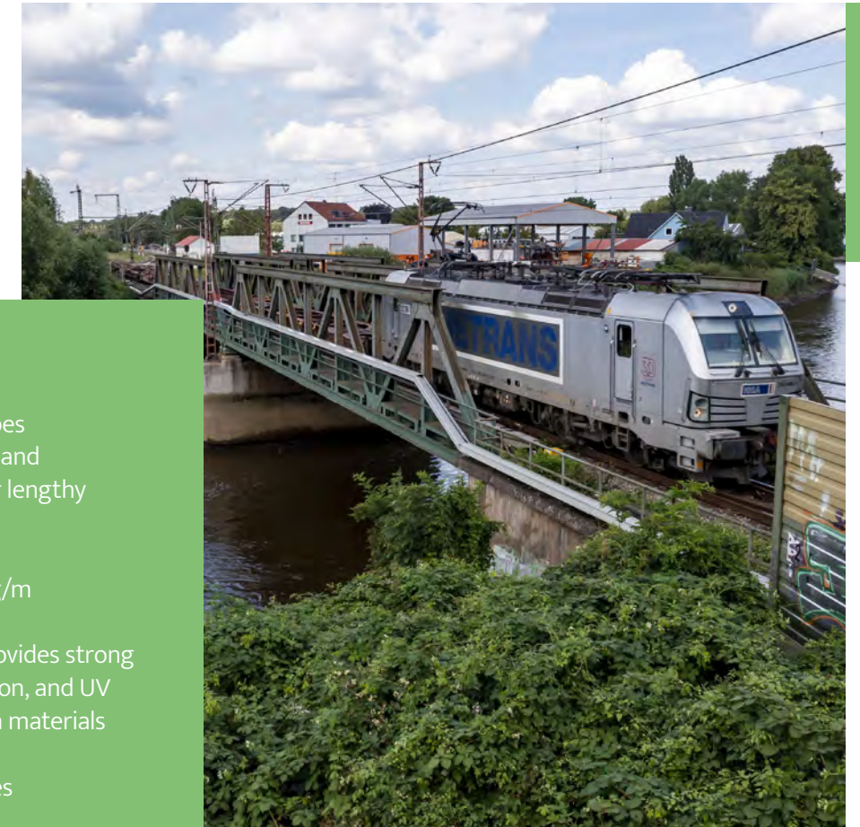
ARCOSYSTEM® safely clamped to a lengthy steel railway bridge over the River Lesum near Bremen
