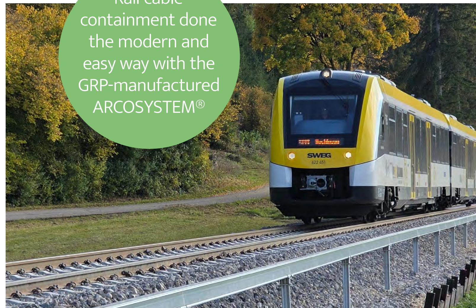
ARCOSYSTEM® rail cable troughing post-mounted trackside at Jungnau in southern Germany
