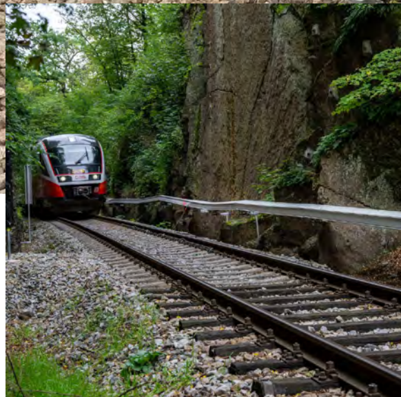
ARCOSYSTEM® attached to a rock wall along the bank of the Danube river in northern Austria
