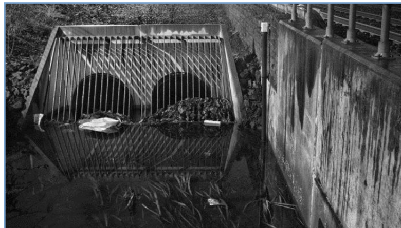
Figure 3: Automated cameras help remote users assess the significance of events such as landslips and rising water levels long before people can visit the site
