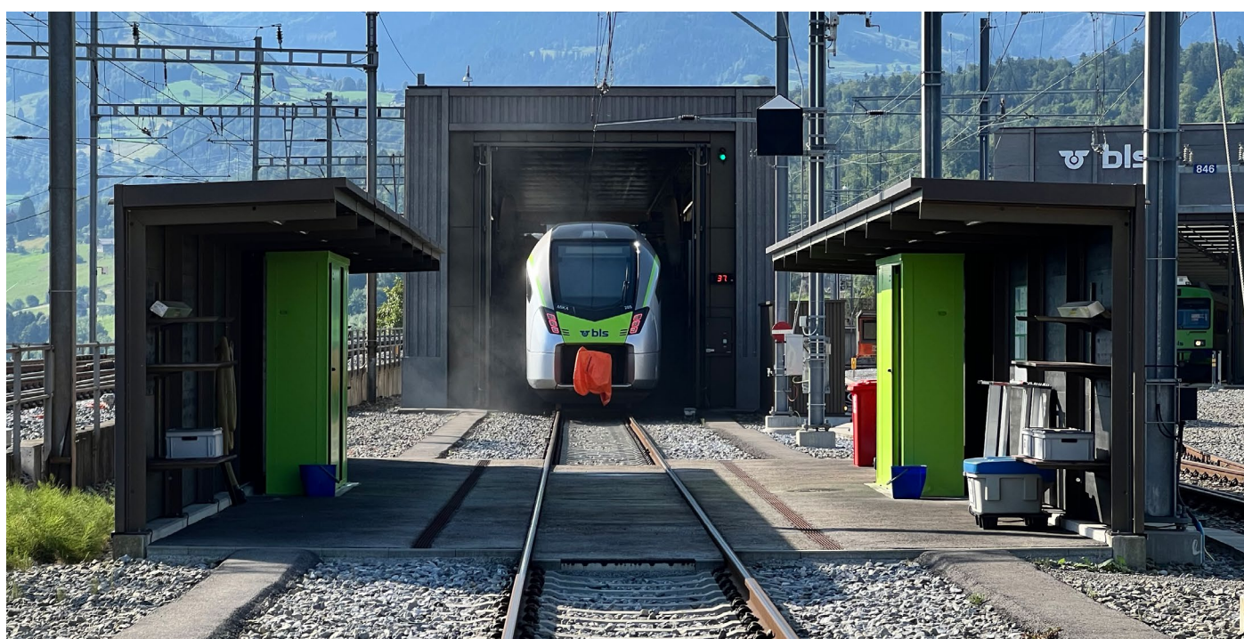
Interior Cleaning Cabinets (aluminium) in Switzerland, Spiez (BLS)
