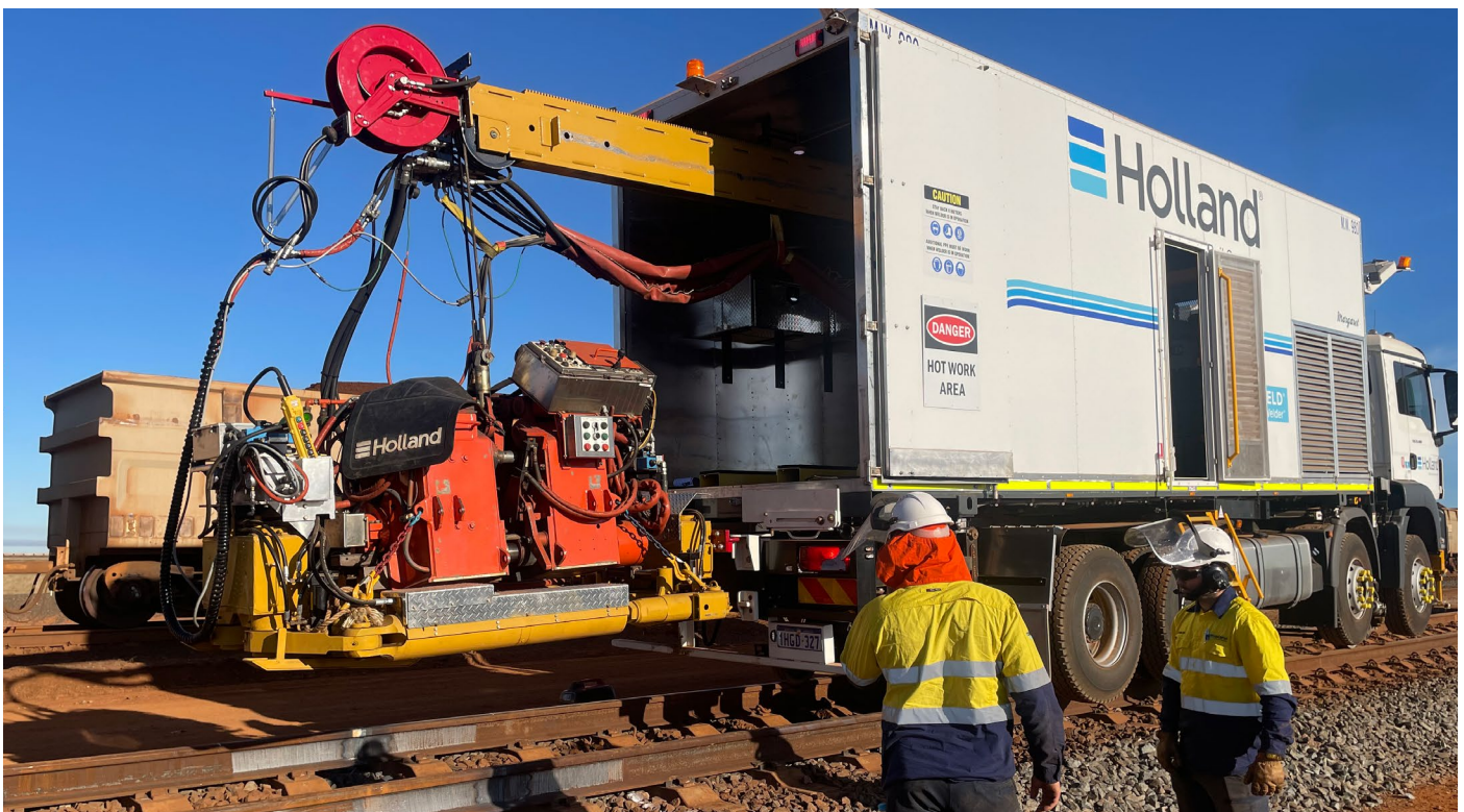
Holland mobile flash-butt welder and puller working in the Pilbara
