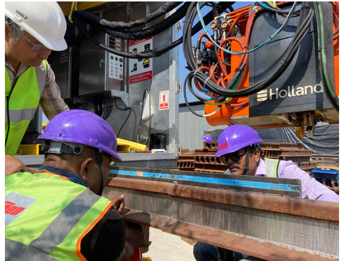
Operators in training during a new flash-butt welder commissioning in India
