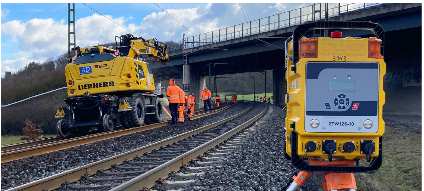
The ZÖLLNER Mobile Radio Warning System consists of light-weight components installed easily at the worksite. The system can be flexibly adjusted using more or fewer warning devices depending on the works carried out, the progress of work and surrounding noise
