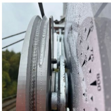
Installation on Sheffield tram 2024
