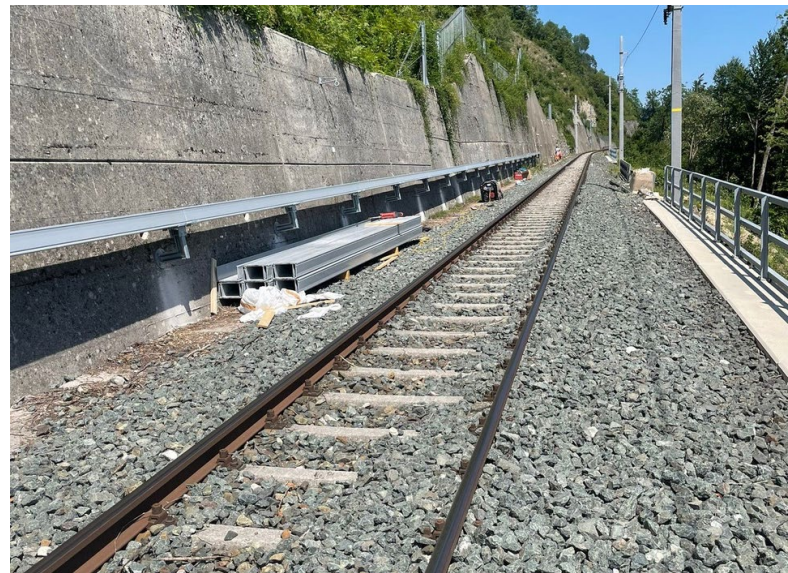
ARCOSYSTEM® safely attached to a slanting concrete wall with the aid of the system's supporting range of bespoke steel bracketry
