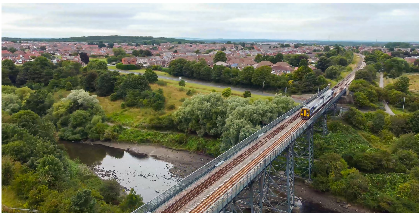
Bedlington Railway Bridge - First trains travel on proposed Northumberland Line route in 2021 © Network Rail
