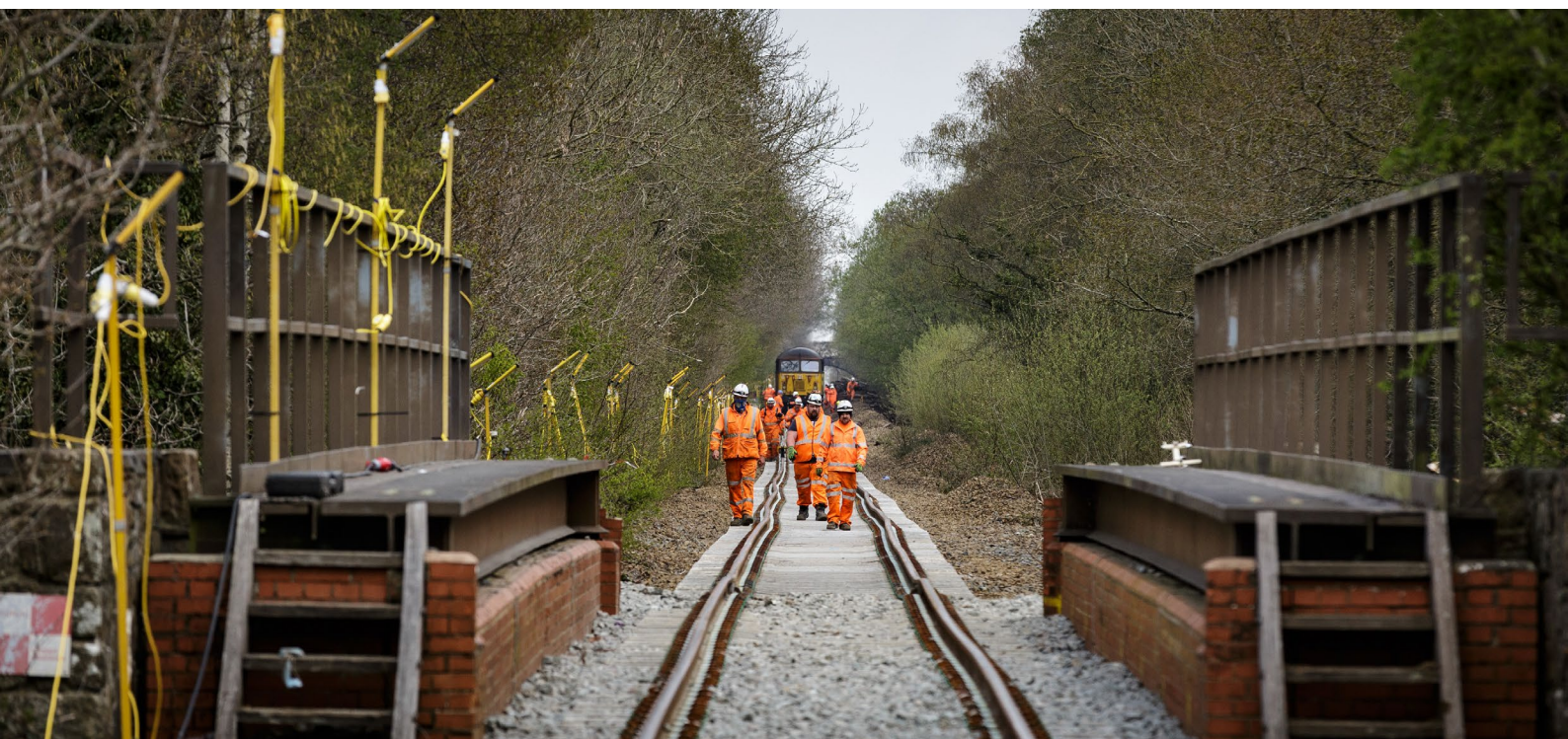
Preparing the Dartmoor Line for reopening © Network Rail
