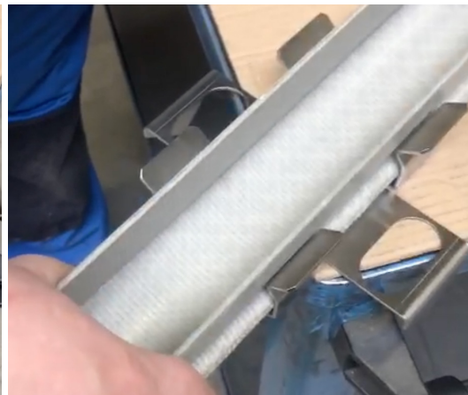
Slotting the troughing into place, activating the bracket to 'click' shut
