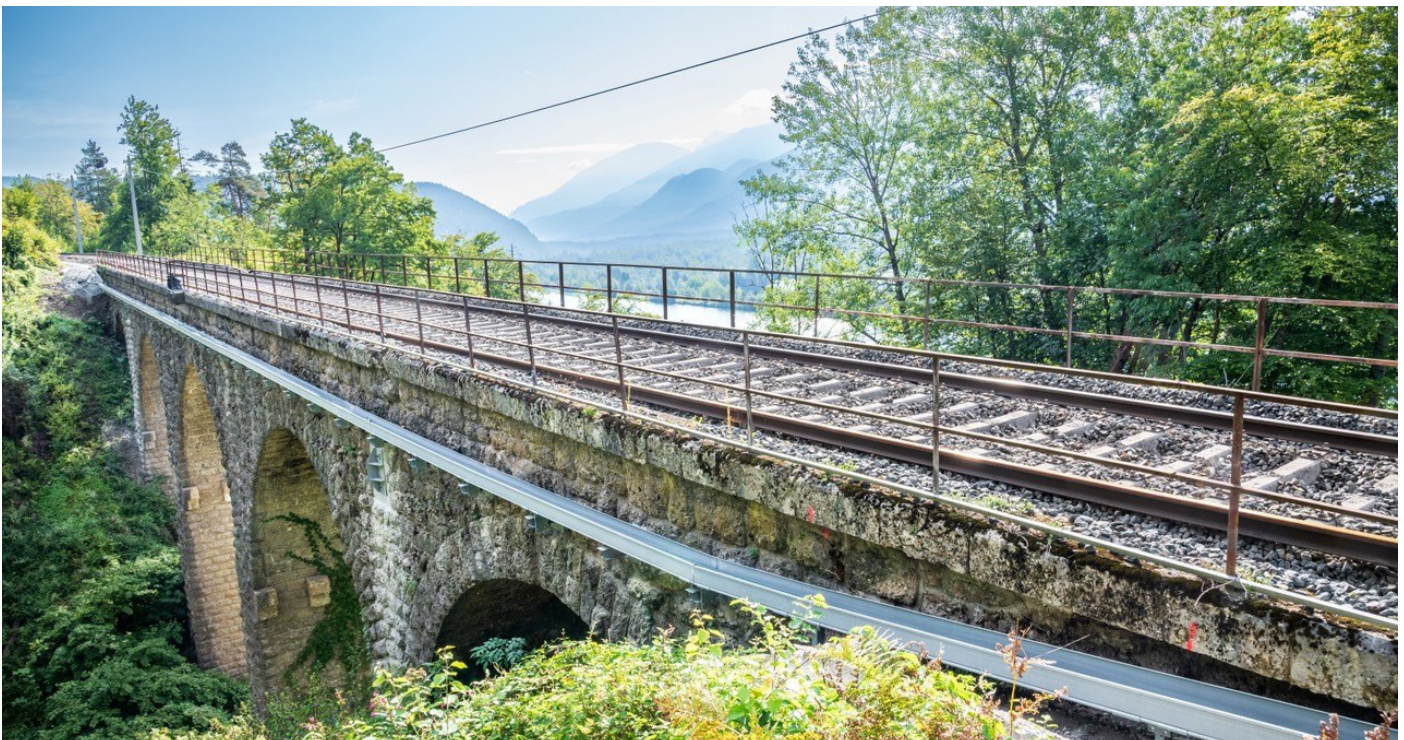
ARCOSYSTEM® troughing attached to the side of a stone bridge near Klagenfurt, Austria
