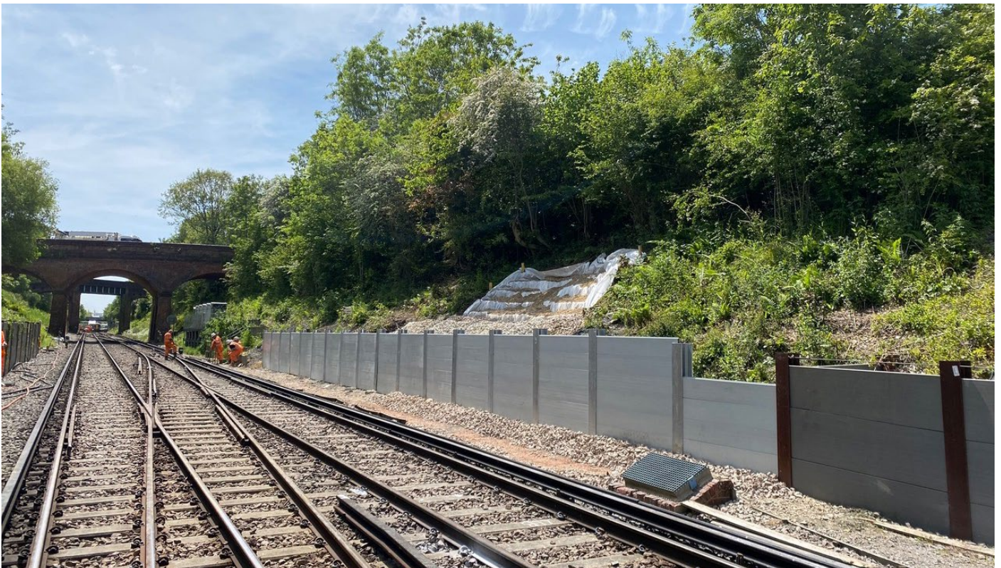
Composite ballast boards from CCS being installed on site
