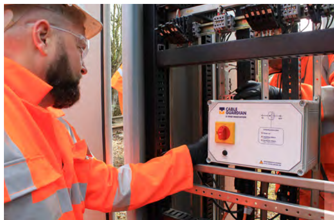
Installation of CableGuardian units can be completed in under an hour without the need to power down
