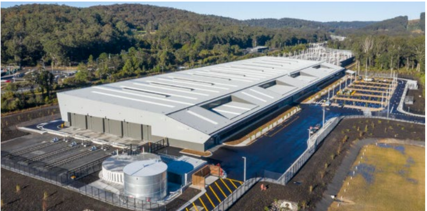
The Mariyung Maintenance Facility in Kangy Angy
