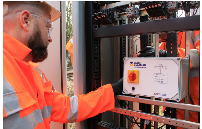
Installation of CableGuardian units can be completed in under an hour without the need to power down
